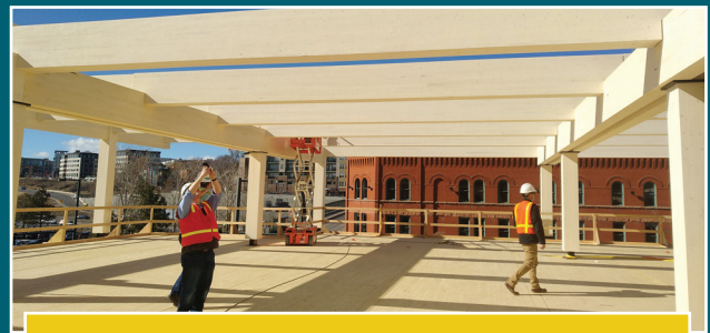
A mass timber building under construction in Denver, Colorado, USA
